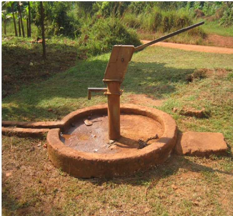
Figure 15: Borehole that consists of groundwater extraction by manual pumping (Photo: C. Prouty)
