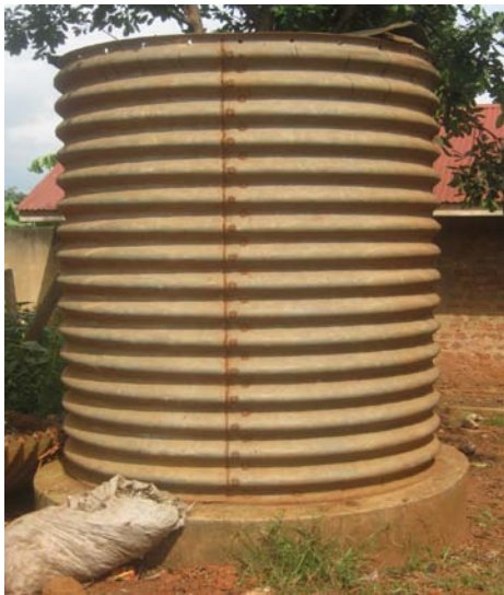
Figure 17: Household rainwater harvesting systems constructed of corrugated metal (left) and plastic (right) (Photo: C. Prouty)
