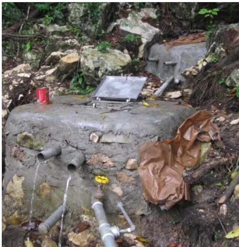
Figure 16: Protected spring water is collected through a springbox and reservoir constructed using metal pipes, cement, and bricks (Photo: C. Prouty)
